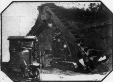
Digging and Loading in Gravel Bank. The broad creeper treads need no planking. The feeding propellers do the digging. One man only—the operator.
